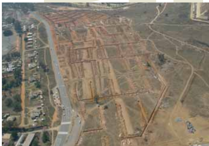
Aerial view of the Pennyville site.
